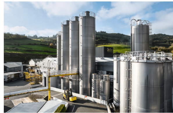
Modernized sites to reduce energy consumption. ↑ Gerflor Tarare plant, France.
